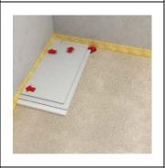
Apply **fermacell** Floor Glue to the edge (2 glue strings approx.  $5 \text{ mm } \emptyset$ )
