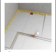
Glue and screw down the continuous fermaceII Powerpanel  $\text{H}_2\text{O}$  Flooring Element – element
