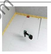
After approx. 24 hours, the hardened floor glue can be scraped off and joints can be filled, e.g. with **fermacell** Powerpanel Surface Treatment.
